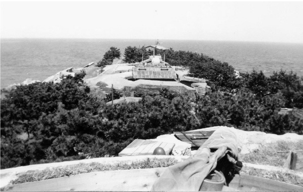
Ft. #2 hilltop view of the fort and of Tokyo Bay beyond. August 30, 1945
